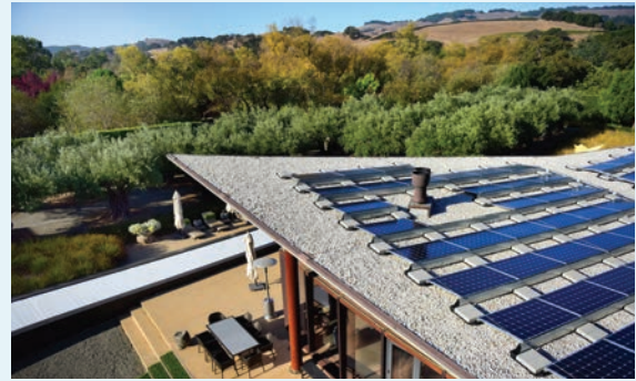
Microgrid at Stone Edge Farm in Sonoma, California, using technology provided by Emerson 96
